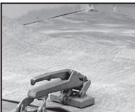
6. After the carpet has been properly aligned into the wet adhesive, the use of stay nails is required to hold carpet alignment until carpet adhesive is fully cured. 24-36 hours.
