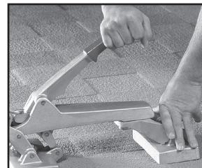
3. Roberts Pattern Matching Stretcher will enable you to "crab walk" the carpet pattern into proper alignment. As pattern distortion can vary in every piece of carpet, it will be necessary to "crab walk" the pattern in multiple locations across the breadth of the distortion to achieve proper pattern alignment.
