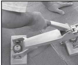
5. Match the pattern at the midpoint of the seam's length. Work from the seam's midpoint to the seam's ends. Bring the pattern into register using the stretcher.
