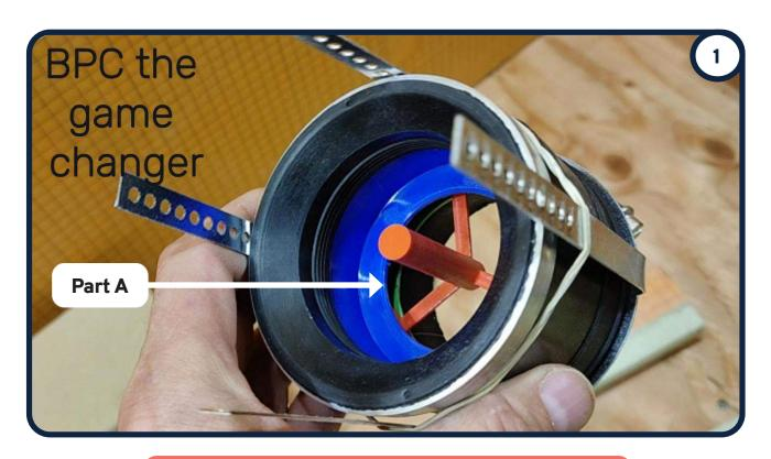
Do not remove the red "Blocking Spider" (part A)
