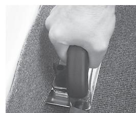
3. Move the trimmer in the opposite direction to complete the cut at the corner.
