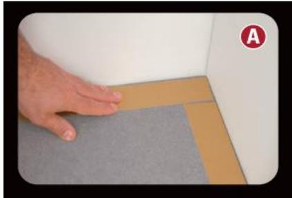
The installation surface should be clean, dry, and debris free. Apply **MAX GRIP** tape liner side up. Press the tape strip firmly to the floor / surface (see A). Firmly adhere the first few inches, and then unroll a foot or two at a time, letting the tape lay over the substrate. Apply firm pressure for a secure bond in place. **Do NOT apply on top of finished flooring such as carpet, laminate or wood flooring as permanent damage may occur.**
