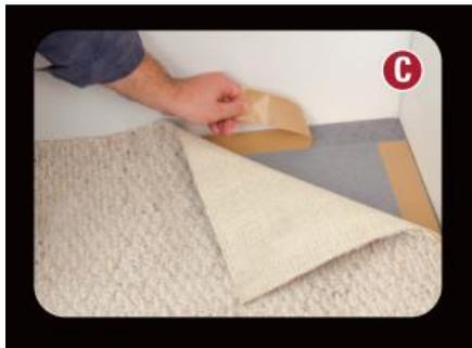
Once flooring is in place, roll back carpet to expose the **MAX GRIP** Tape. (see C). Remove the liner in sections. Once each section is removed, use a weighted hand roller to secure the flooring into the tape. For seams, apply strip under pre-cut seam, remove liner and press both sides of the seam firmly into the adhesive. Finish by rolling the seam with a weighted hand roller.
